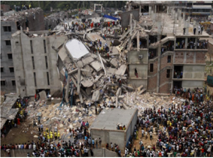
The collapse of the Rana Plaza in Dhaka, Bangladesh.
